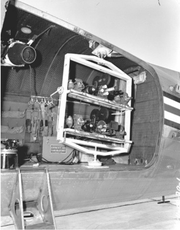
Exterior of camera installation in C-47, JANGLE 4.1
